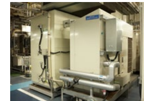
JIZAI HEAT installed at the Rinkai Factory
