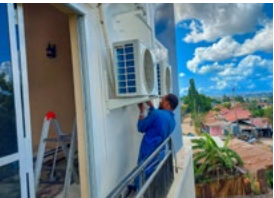
Installing an outdoor unit at a house
